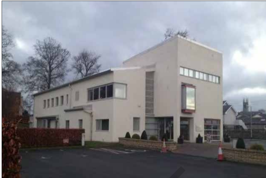
Figure 5.3: Navan Education Centre where Open Days were held Following the Publication of the Final Re-evaluation Report and Preferred Project Solution Report .
